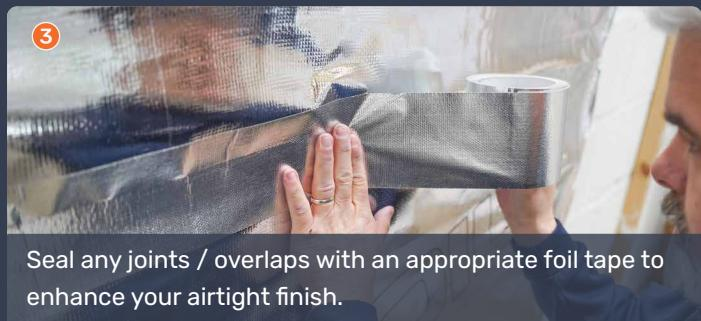
Seal any joints / overlaps with an appropriate foil tape to enhance your airtight finish.
