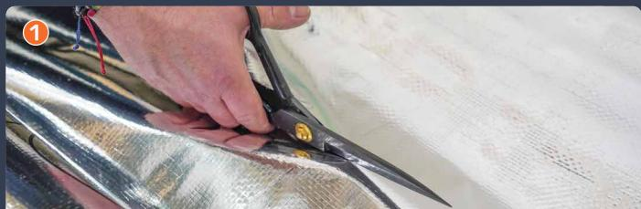
Measure the project area, then cut the insulation to the measured size using heavy-duty scissors or a utility knife.
