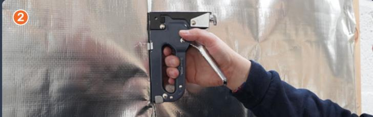
Secure the product to the surface with a staple gun. When installing to hard surfaces, use timber battens.
