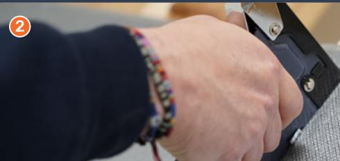
Secure the product to the surface with a staple gun. When installing to hard surfaces, use timber battens.
