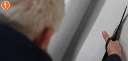
Measure the project area, then cut the insulation to the measured size using heavy-duty scissors or a utility knife.
