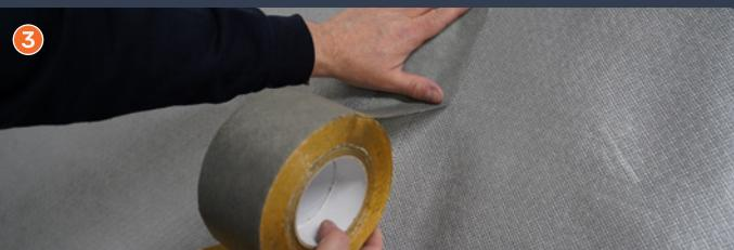
Seal any joints / overlaps with an appropriate foil tape to enhance your airtight finish.
