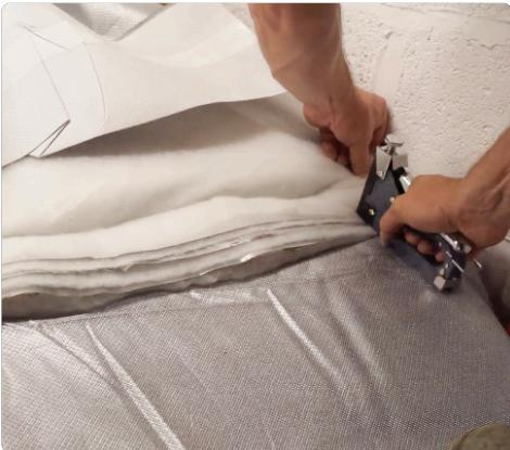
Properly securing the insulation is essential. To do this, you should first compress the SuperFOIL and then staple it to the rafters using appropriate staples (refer to page 2 for staple sizing).
