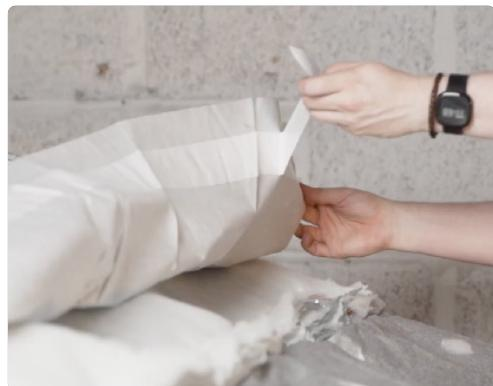
Sealing the 100mm overlap between runs is vital to the airtightness of the installation.
