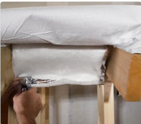
At the wall plate you should ensure that the insulation layers (beneath the breathable membrane top layer) overlap it slightly.
